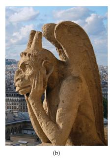
▲ FIGURE 18.8 Damage from acid rain. The right photograph, recently taken, shows how the statue has lost detail in its carvings.
